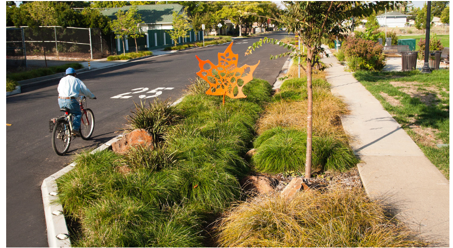
A bulb-out incorporating green infrastructure to manage stormwater and enhance the streetscape.
