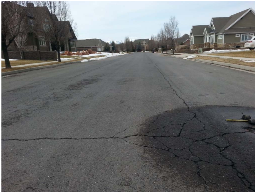
Figure 2. Woodland Drive (Segment 75) - Typical Non-Structural Durability Distress
