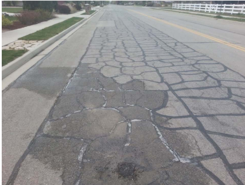
Figure 3. 11200 North between 4930 West and 4800 West (Segment 180) - Typical Structural Distress
