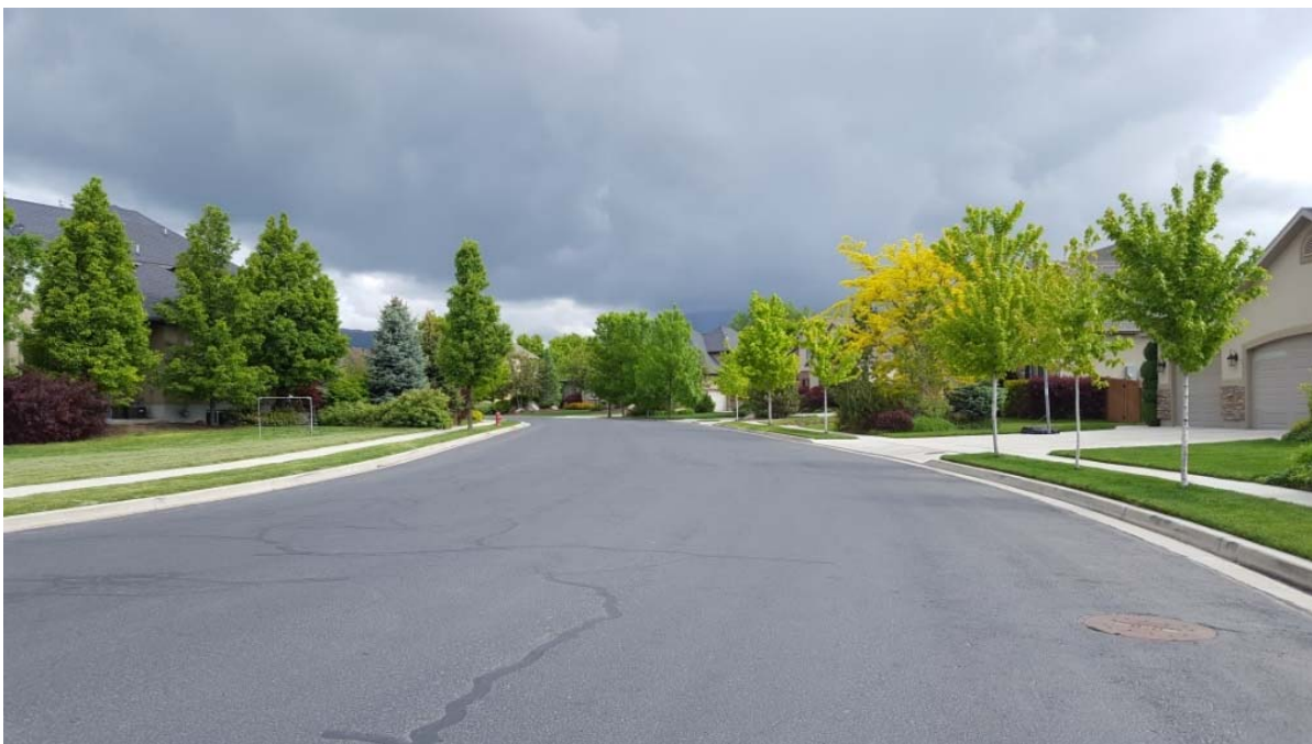
Figure 4. Canterbury Drive - Typical Durability Repairs of Crack Sealing and Sealcoating.
